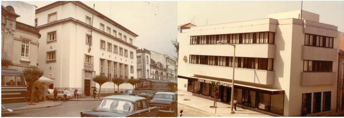
Fig. 47 – The Viana do Castelo branch of Caixa Geral de Depósitos after the alterations (left) and the new version of the building in 1983 (source: Caixa Geral de Depósitos).
