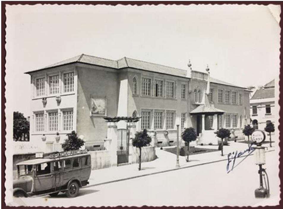
Fig. 40 - View of the school with the fuel pump in the right-hand corner of the image (source: private collection)
