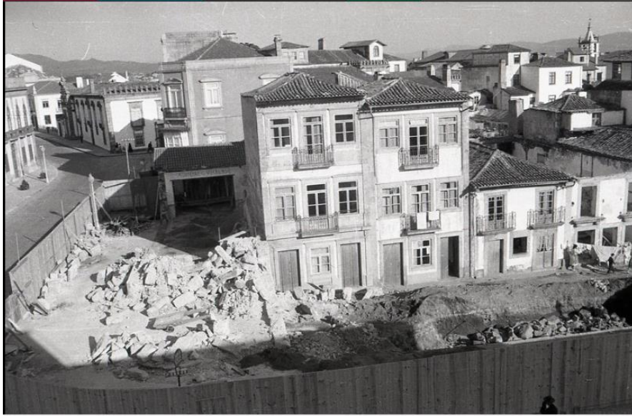
Fig. 34 – The corner before demolition started (Source: _)
