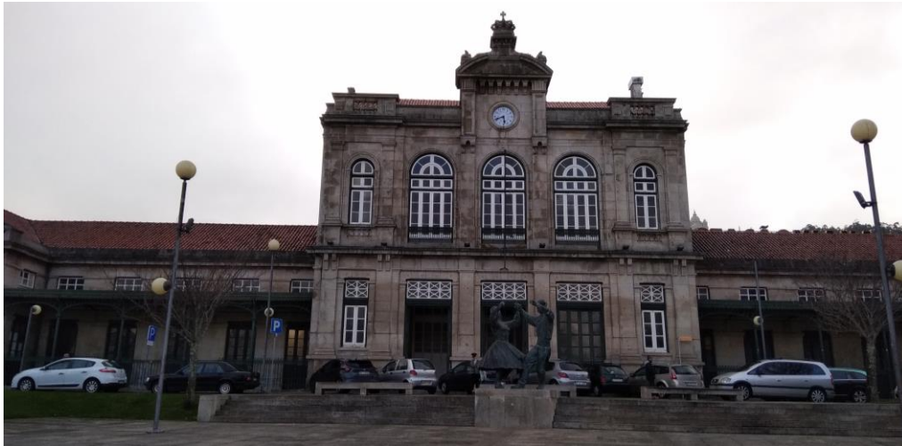
Fig. 6 The railway station of Viana do Castelo (source: author)
