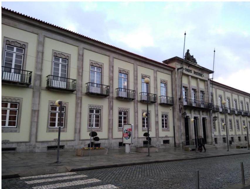
Fig. 38 – The Courthouse the now occupies the corner of the main avenue (source: author).
