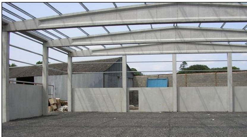
Figura 7 – Structure 17, M50 Dublin
