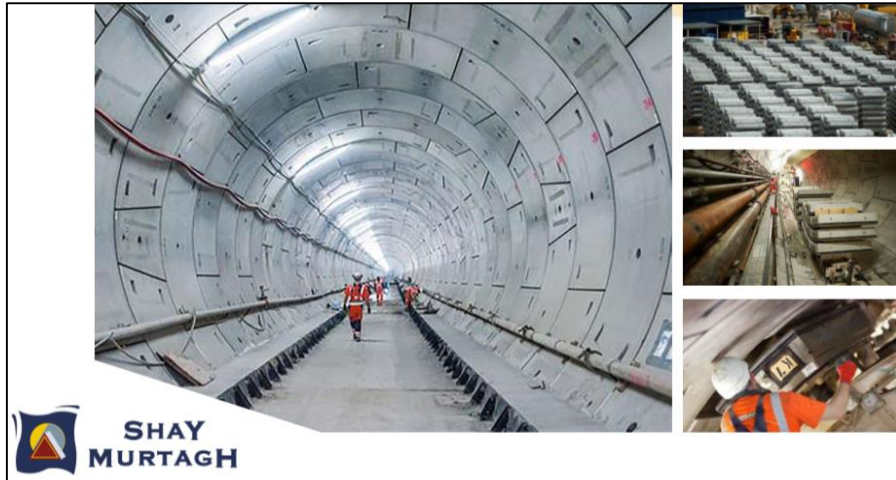
Figura 6 – Crossrail C310, Thames Tunnel, Londres
