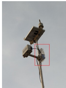
Figure 6 - Weather station and LoRa device
