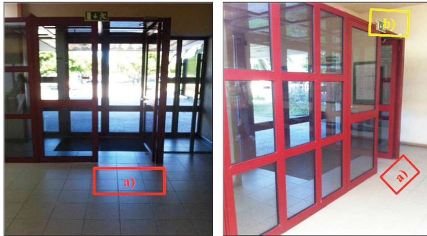
Figure 10.6. ESTG-IPVC's main entrance: a) location of the carpet with the respective piezoelectric; b) location of emergency exit lighting
