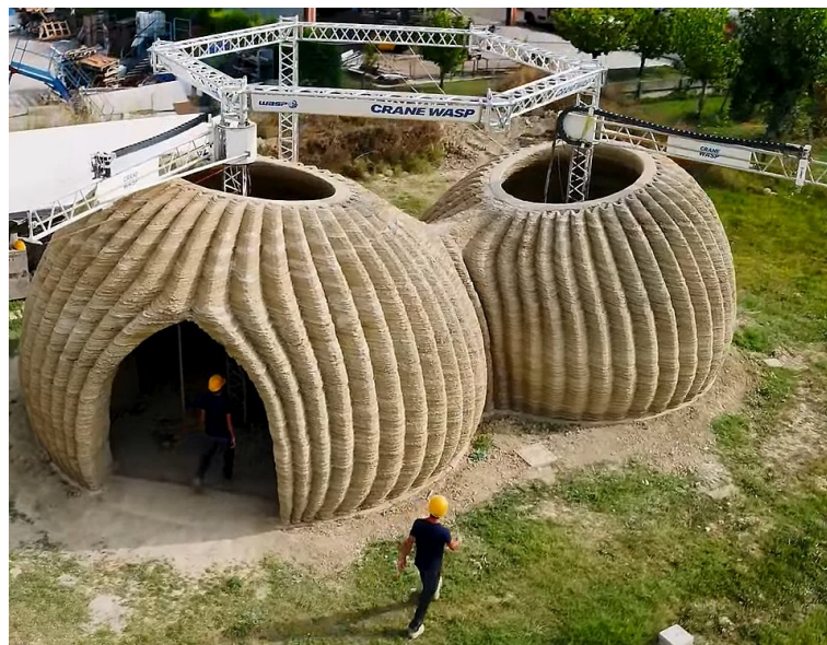
Figure 21. The Tecla houses that have been 3D-printed by two large synchronized robotic arms. Licensed under the Creative Commons Attribution 2.5 Generic license [130].
