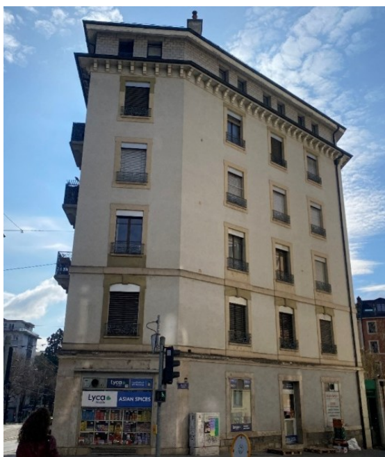
Figura 20 - Fachada Norte do imovel (Inpto Engineering)
